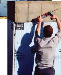
Sealing foam insulation board on outside walls
